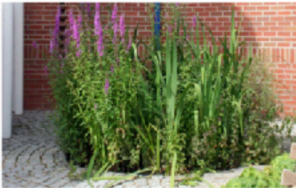
Image: an unlined raingarden within 5m of a building
